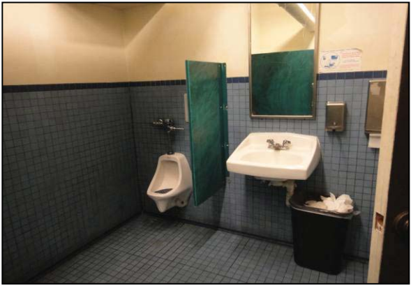
Basement men's room
