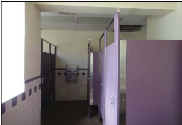
1 st floor women's room
