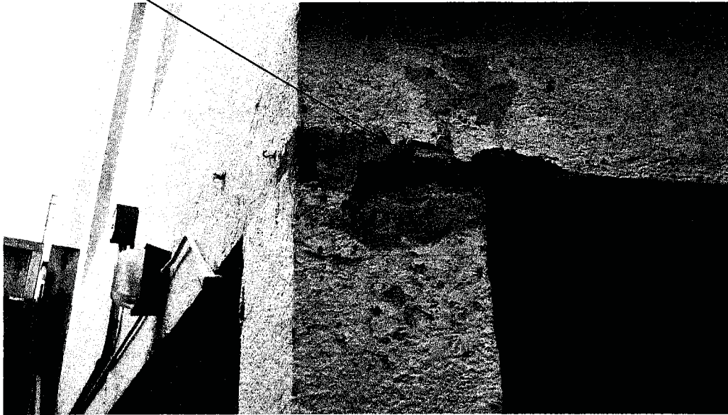
STAGE ADDITION CONCRETE COLUMN SPALLING
