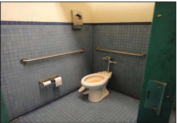
Basement men's room
